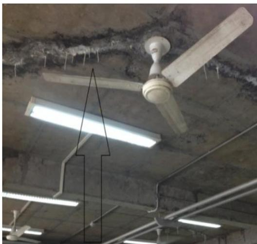
Figure 1: White scaling under roof slab
