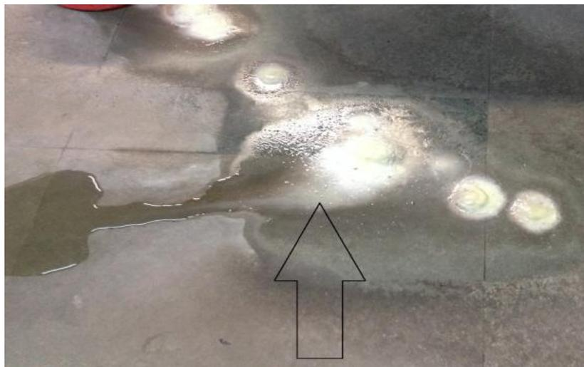
Figure 3: Dropout of whitish bloom material on floor
